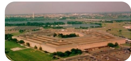
Pentagon Renovation after 9/11
